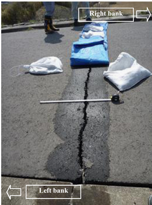
Photo 4. Cracking in the stream direction on the crest of Kejonuma Dam.
