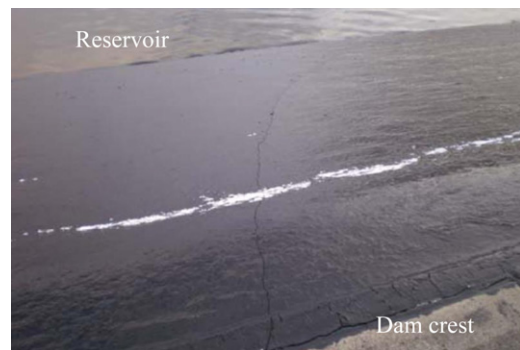
Photo 5. Cracking of the asphalt facing of the Minamikawa Saddle Dam.
