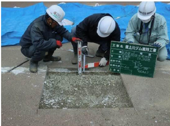
Photo 2. Crack depth analysis at Surikamigawa dam.
